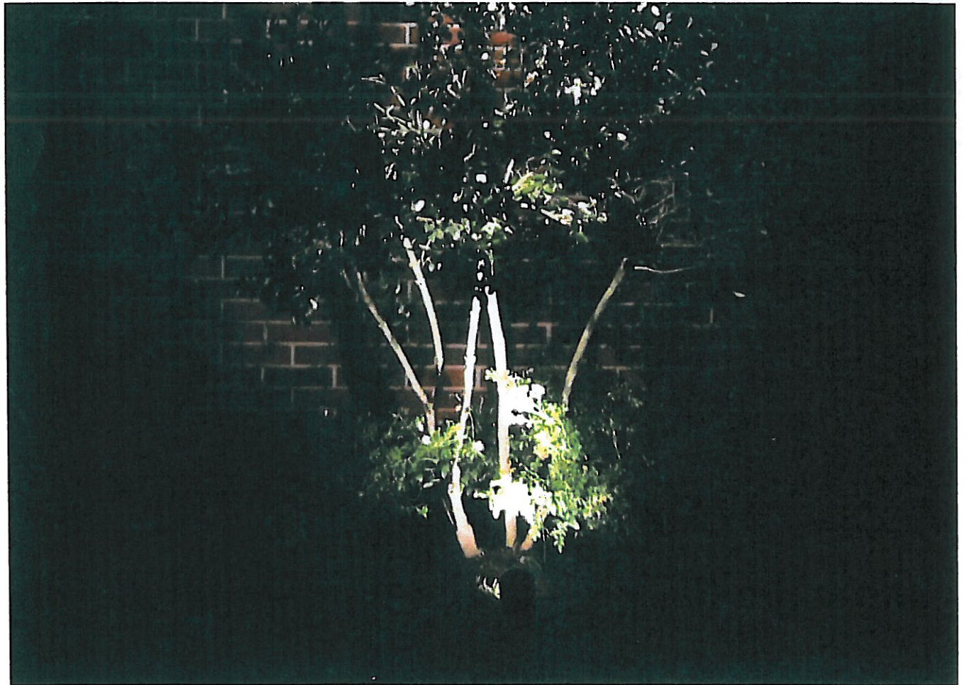
Acceptable style of low voltage accent lights that do not show the light source
