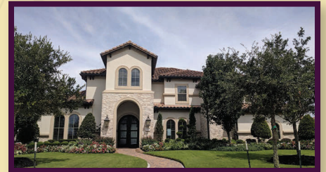
Section 3: 5043 Water View Bend
